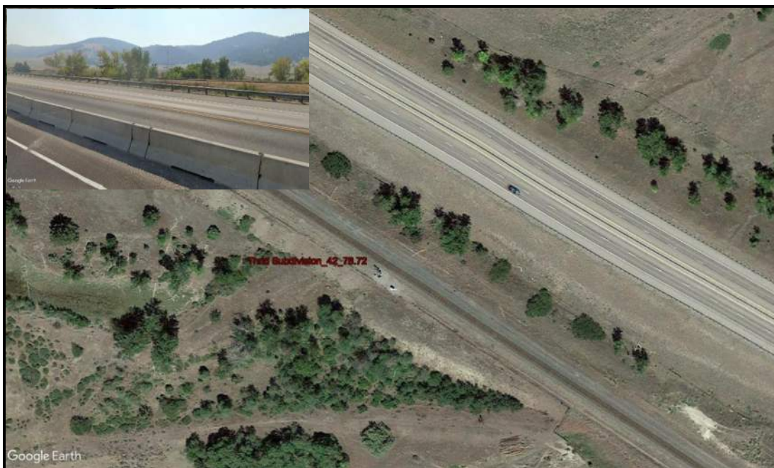
Figure 8. Overview of the proposed location for Third Subdivision_42_76.72.
